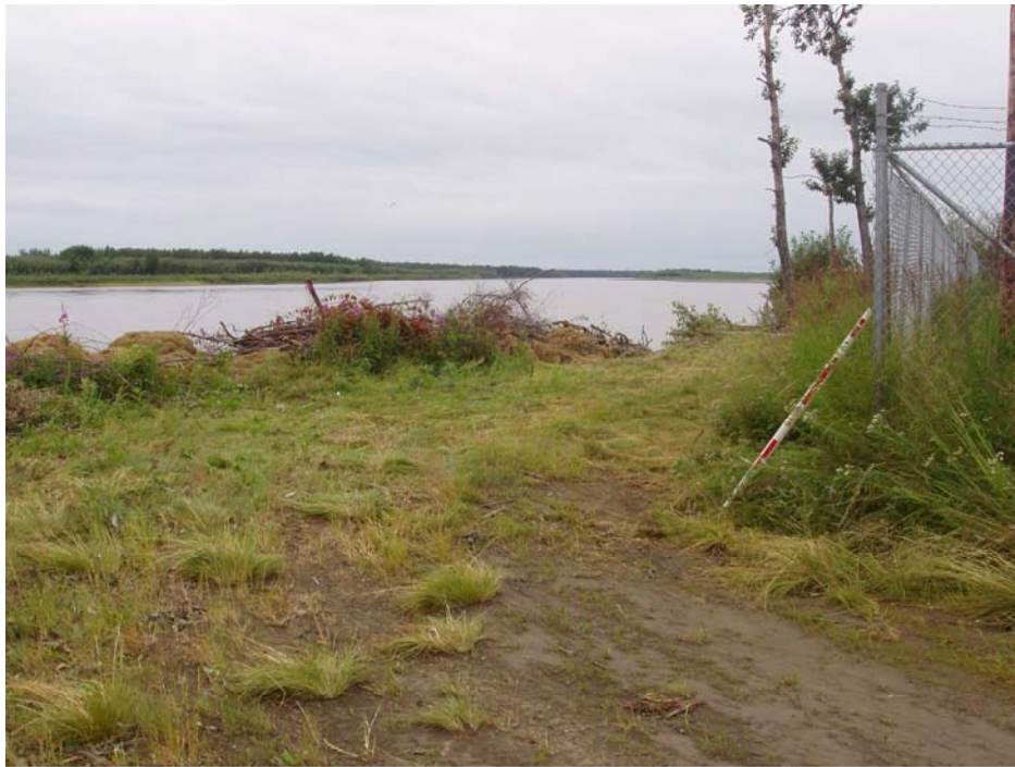
Photo 1. Perimeter fence around old tank farm, upstream corner 25.0' from top of bank. Downstream corner <1' from top of bank.
