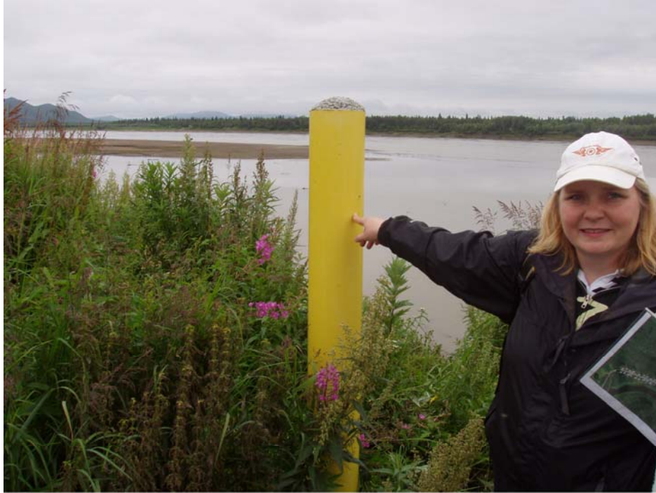
N 61° 30.727' W 160° 21.605' Lower Kalskag P1011212 Photo 2. Bollard protecting school filling point looking towards the river, 7.0' to the top of bank.
